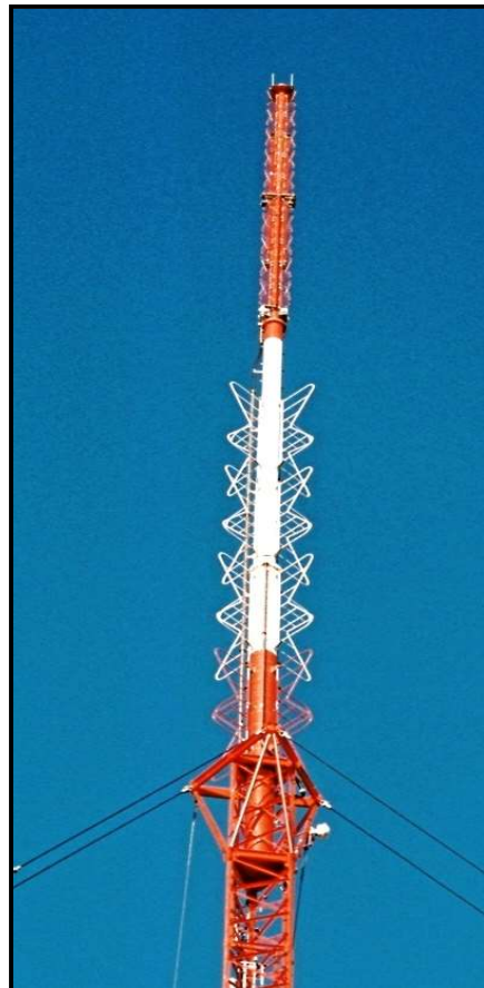
High-Power Channel 13 and Channel 3 Stacked Antenna Installed on the Tower in Bend, Oregon
