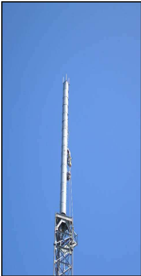
Channel 13 and Channel 41 High-Power DTV Broadcast Antenna Being Installed on Mt. Mansfield, in Vermont
