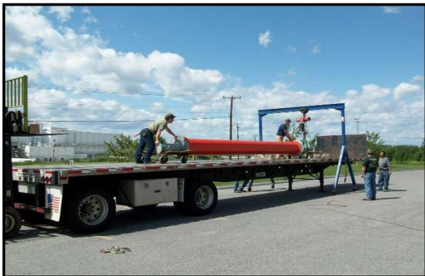
Elliptically-Polarized Channel 8 DTV Transmitting Antenna, Being Shipped to Sandia Crest, NM
